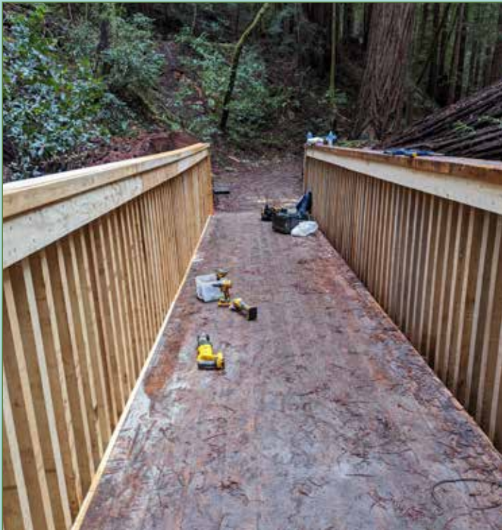
Bridge is done. Thanks to Mike Bushue and his team of volunteers.
