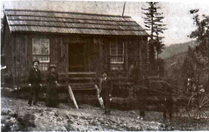
Sunday at Rider's Mill in the Soquel area. A typical woodcutter's cabin with board-and-batten siding and a split shake roof.
