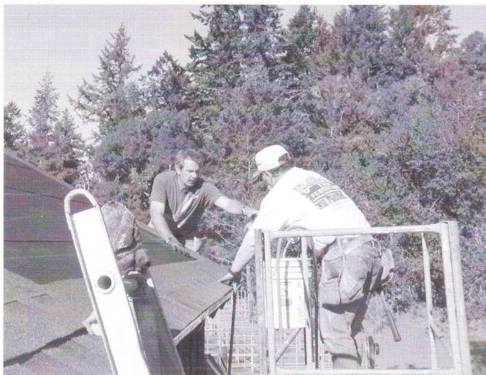
Volunteers replace the barn roof in Fall 2004
